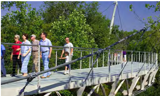
A suspension pedestrian bridge provides safe access surrounded by nature.
