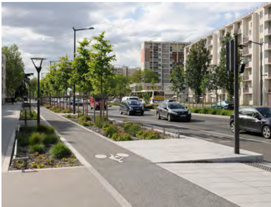
An elevated and protected bike lane provides a safe way for bicyclists to get around without having conflicts with cars or pedestrians.
