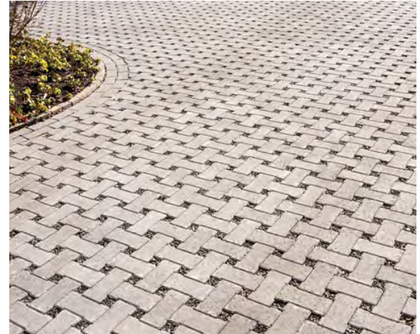
A unique paving treatment provides an interesting texture and is pervious to allow for water to penetrate.
